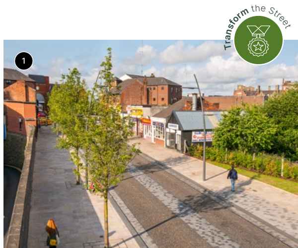
A 6m carriageway with a raised median, breaking up the visual width of the road to calm traffic (Photo: Preston City Centre)
